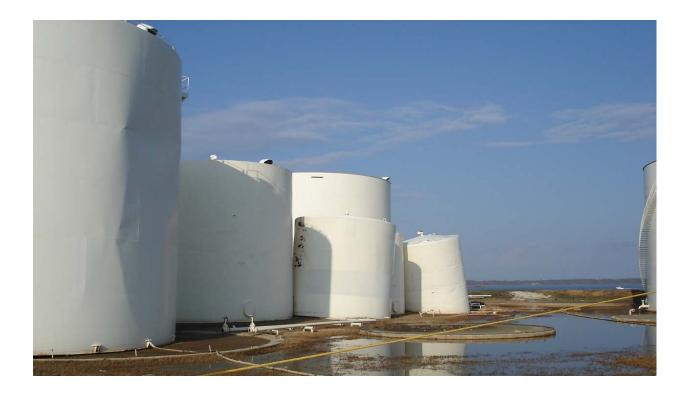
**Figure 3:** Displaced oil tanks at the Munro MP Terminal in Biloxi. Some tanks were displaced more than 40 m and even crossed the spill controlled embankment built around the tanks.
