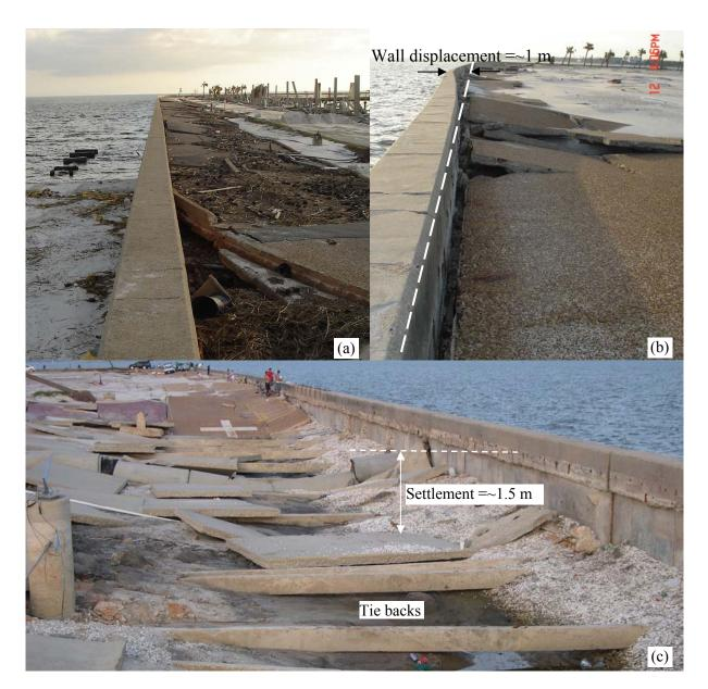
**Figure 1:** Retaining wall failure in the Broadwater Beach Marina. (a) The 450-m long east retaining wall suffered no damage; however, the fill under the pavement eroded and the pavement settled about 0.7 m. (b) The 240-m south retaining wall rotated more than 1.0 m towards the Gulf of Mexico. (c) The backfill for the south wall eroded, the pavement settled and the tie backs failed.
