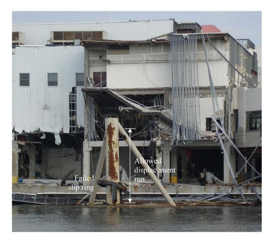
Figure 4: Anchor system and failed slip rings of the Grand Casino barge.
